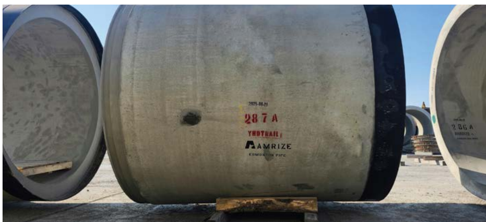
2500 mm Diameter micro tunneling pipe ready to be loaded and installed under the Yellowhead Trail.
