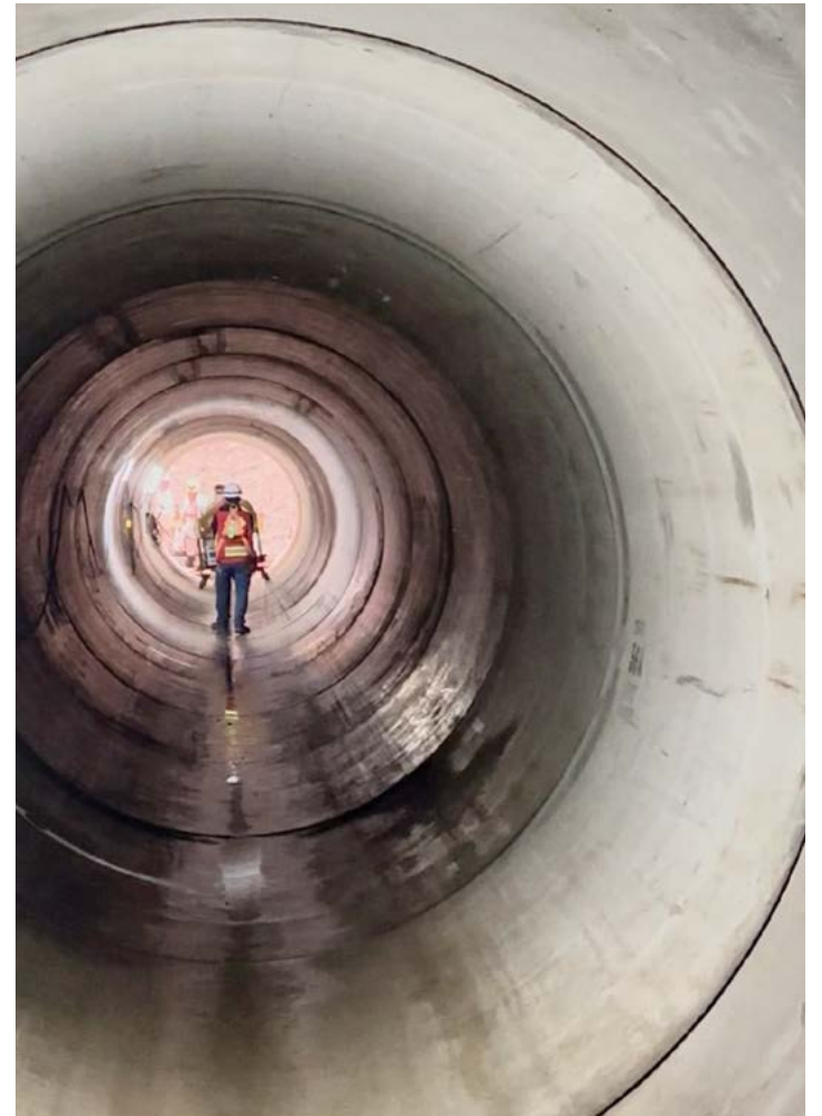
Finished 2500 mm Diameter micro tunneling pipe.
