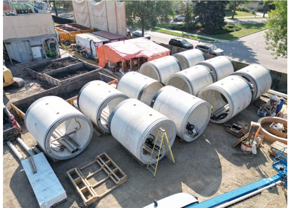
2500mm diameter microtunneling pipe stockpiled at the launch shaft site.
