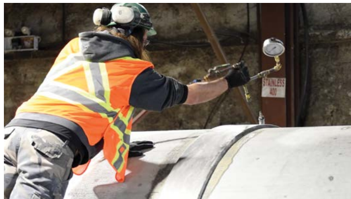
Testing of Concrete Pipe Joint using "Deep Seal" gasket
