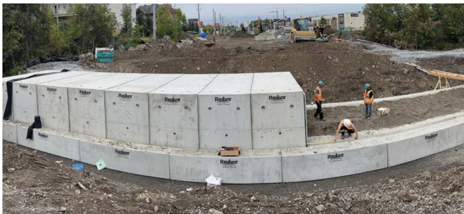
Side view of culvert installation
