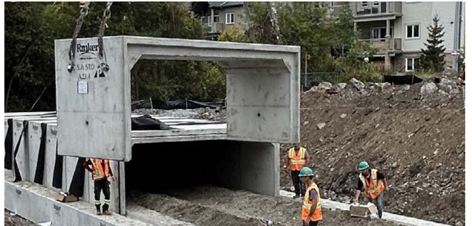
Front view of culvert installation
