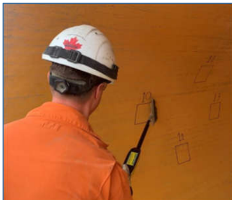
Figure 5: Spark Testing of Liner
