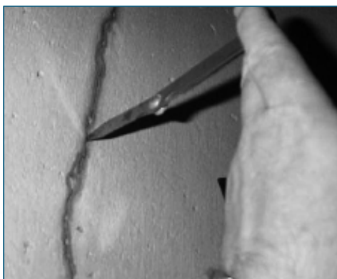
Figure 3: 0.3mm Leaf Gauge to Check Crack Width
