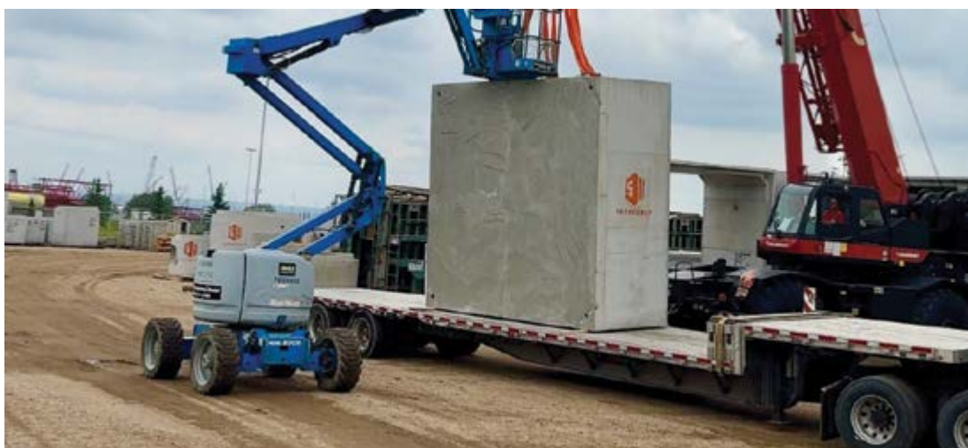
Fire suppression tank segment being loaded for shipping
