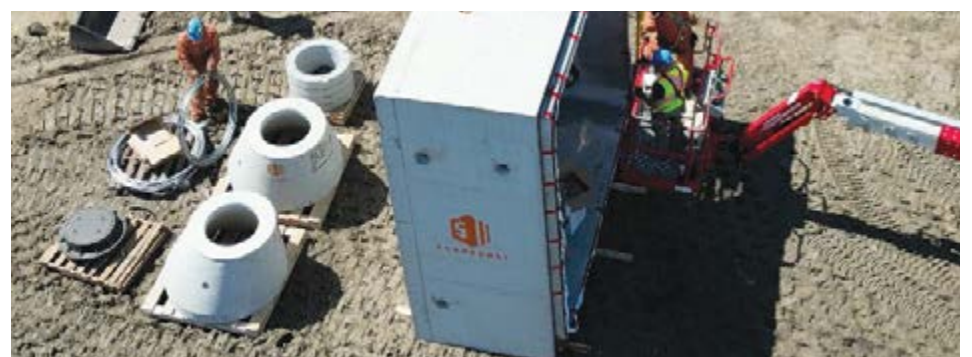
Tank segment being prepared for installation
