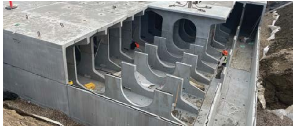
View of internal structure
