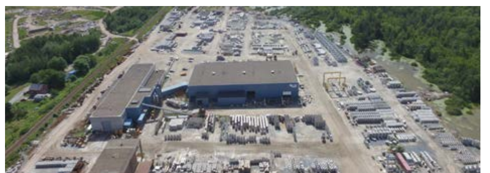
Overhead view of Shaw Precast Solutions Manufacturing Facility located in Lantz, NS.
