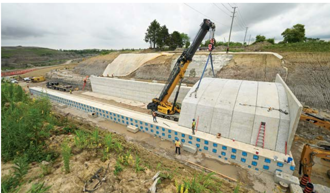
Installation of arch segments
