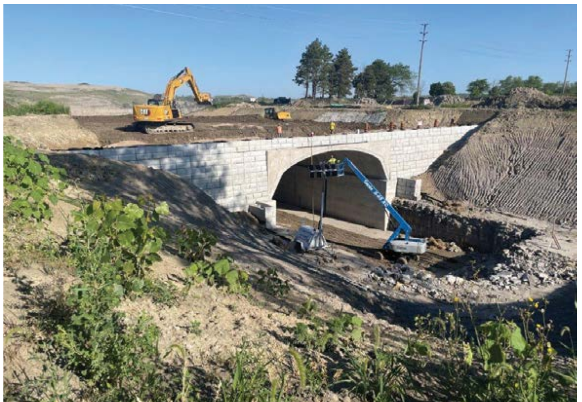
Backfilling of headwall
