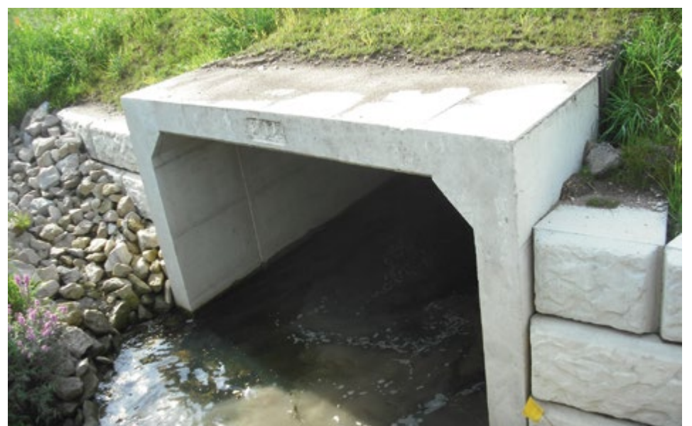
South Boundary Drain - 3.0m x 2.3m precast box culvert
