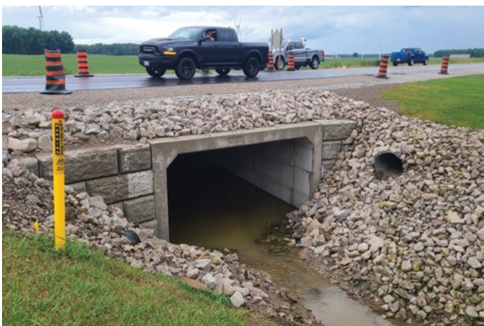
McPherson Drain - 3.6m x 2.4m precast box culvert
