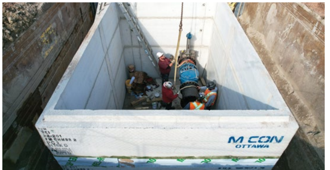
Close up of chamber installation
