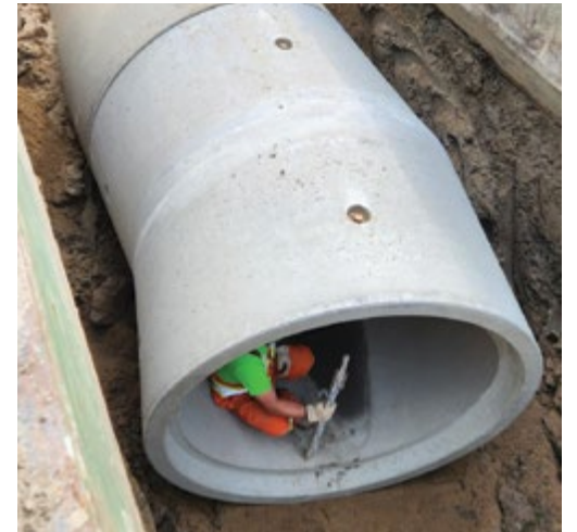
Reinforced Concrete Pipe with custom bend
