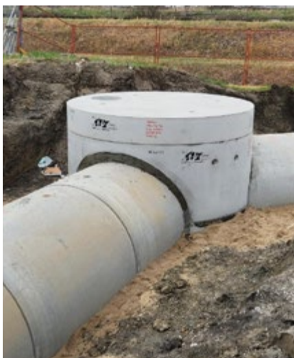
Typical pipe to MH connection
