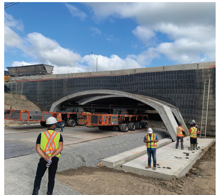
Phase 2 culvert install begins with uninterrupted traffic flow.
