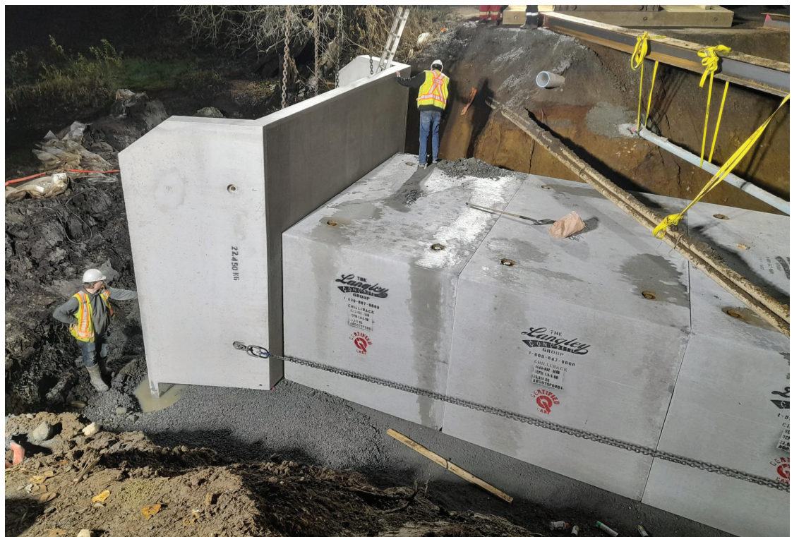
Final installation of culvert structure.
