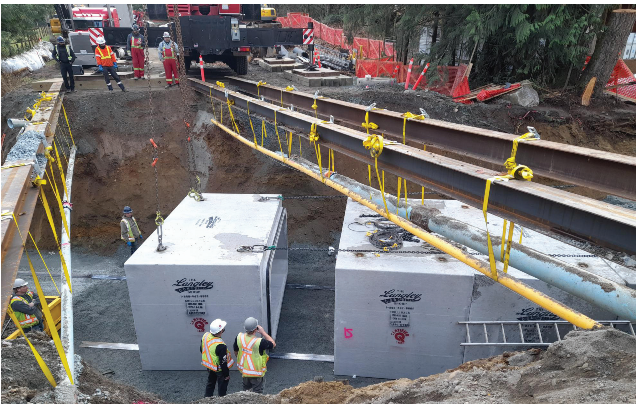
Challenging installation with numerous utilities.
