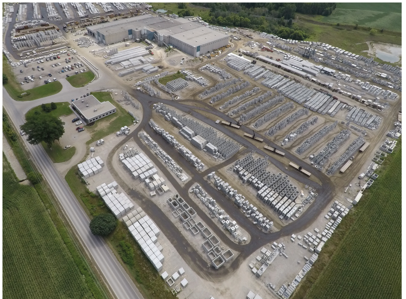
OMNI Precast Manufacturing Facility
