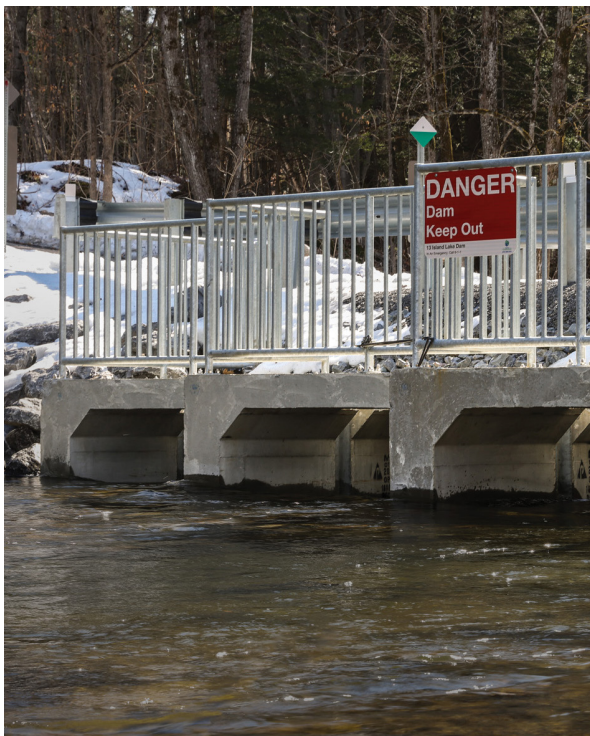
Completed box culvert dam structure.
