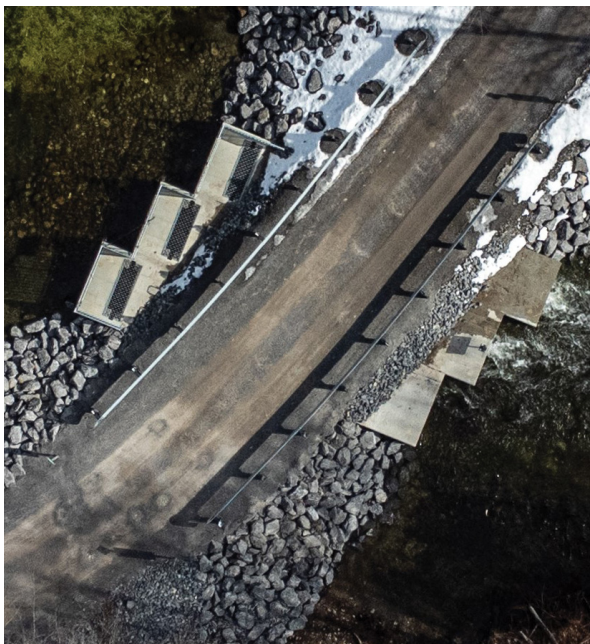
Overhead view of completed box culvert dam structure.
