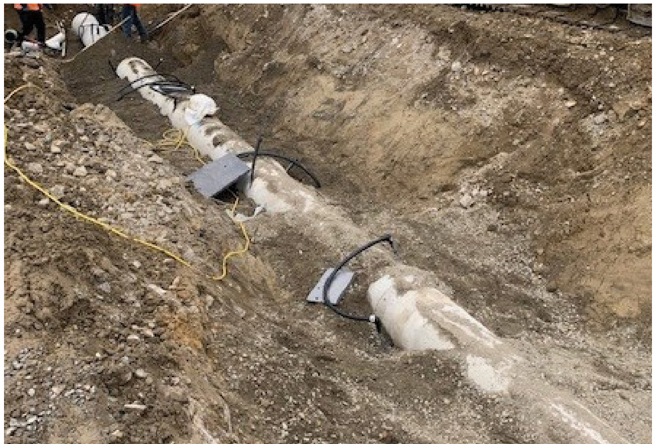
Installation of the specialized reinforced concrete pipe
