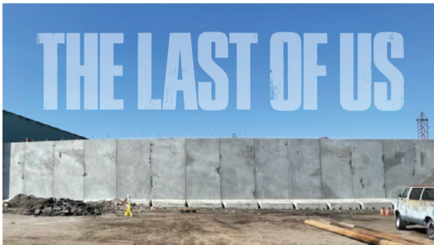
Installed precast structure
