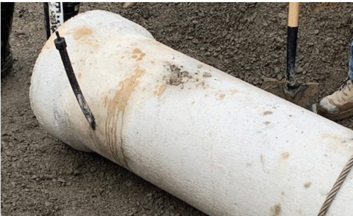
Closeup of reinforced concrete pipe with integral heat exchanger encasement
