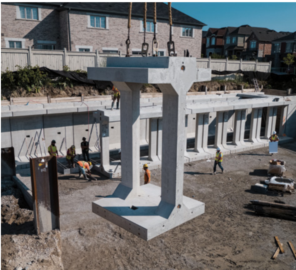
Picture 1: I-STORM being installed
