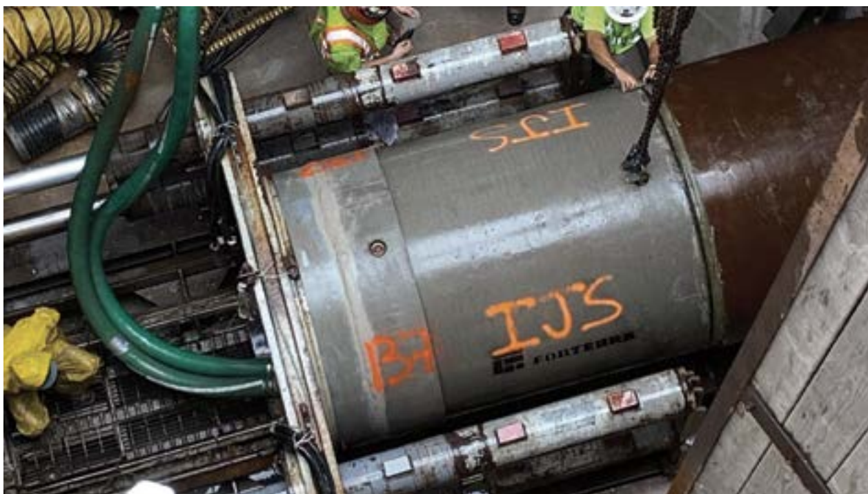
Close up view of microtunneling jacking rig and pipe
