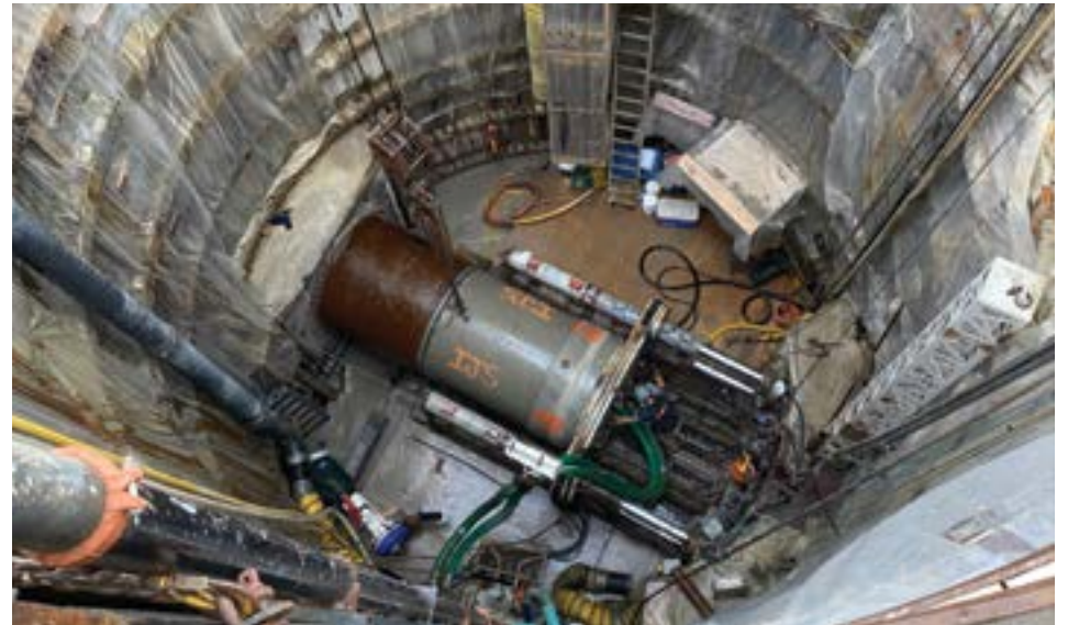
View of launch shaft
