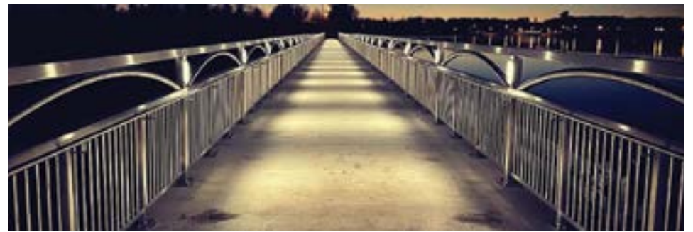
Completed dam walkway
