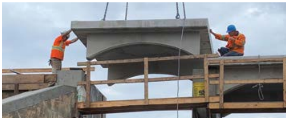
Deck/arch segment lifted into place
