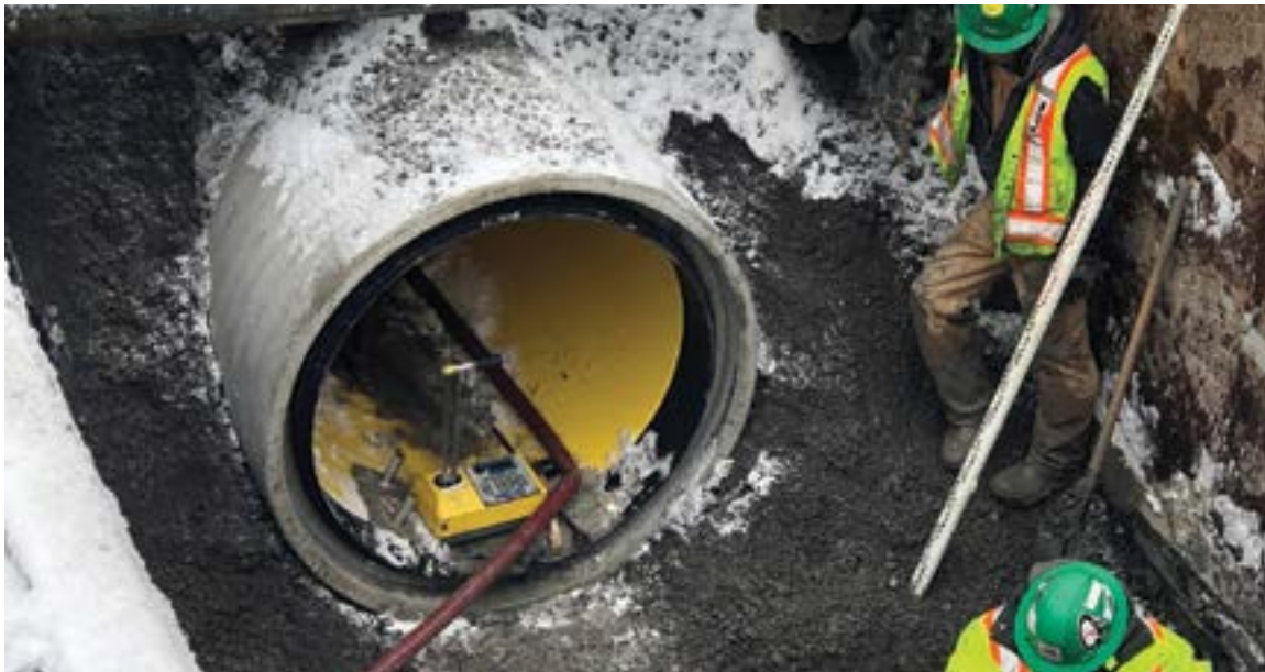
PERFECT Pipe installation
