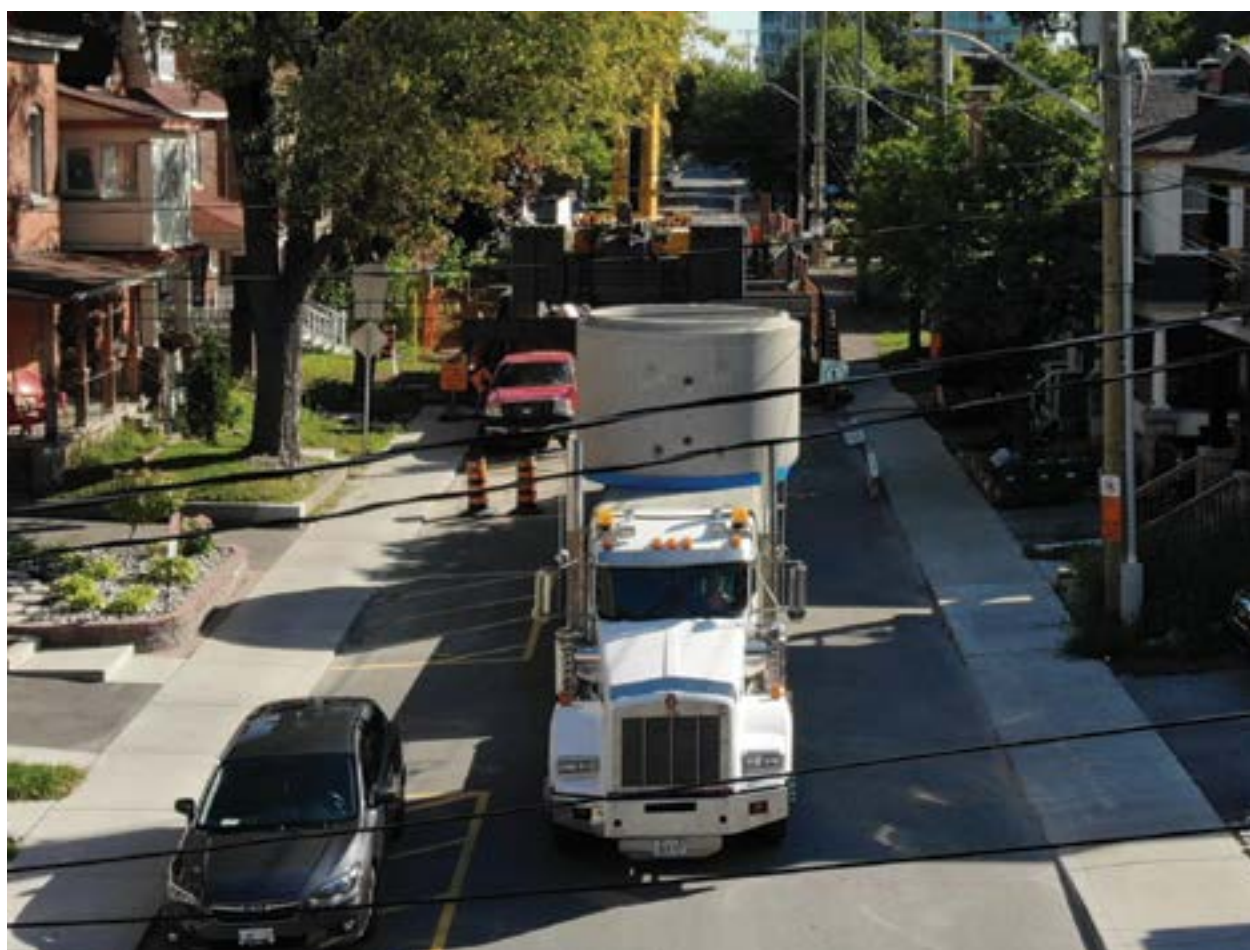
3000 mm ID pipe delivered to the jobsite
