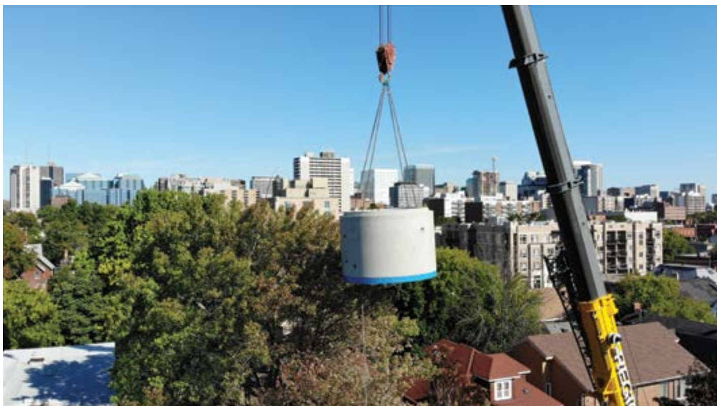
3000 mm ID diameter pipe lifted into place
