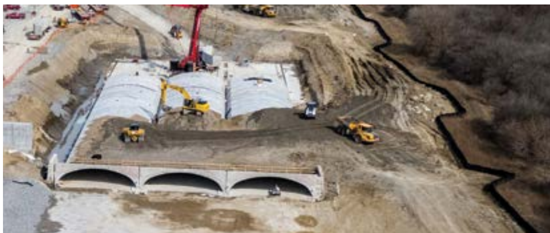
Overhead view of installed precast stormwater structure
