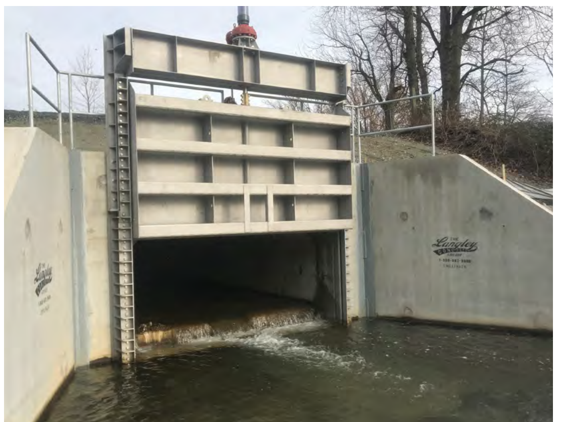
Downstream end with vertical slide gate
