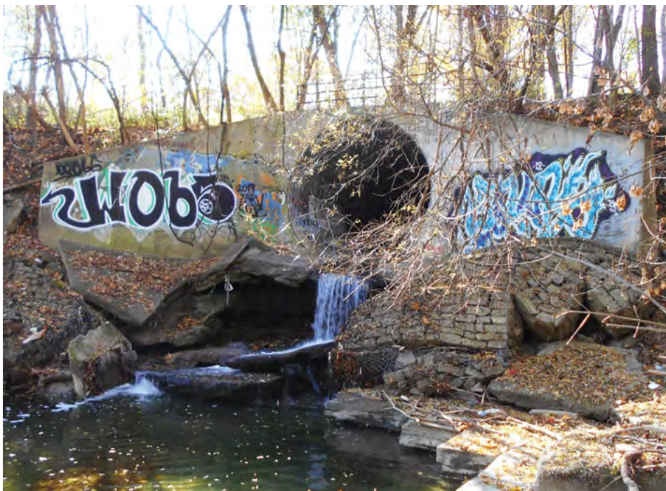
Existing structural plate corrugated steel pipe culvert
