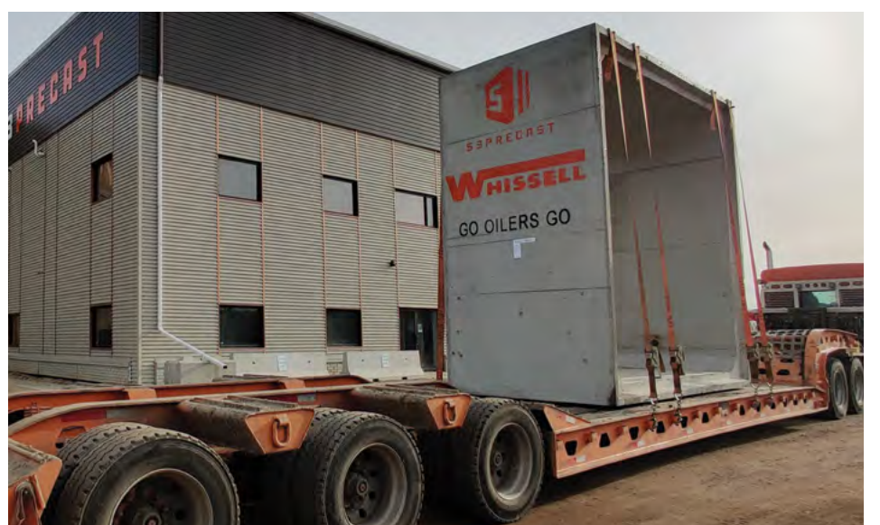
4 m x 4 m box culvert being delivered
