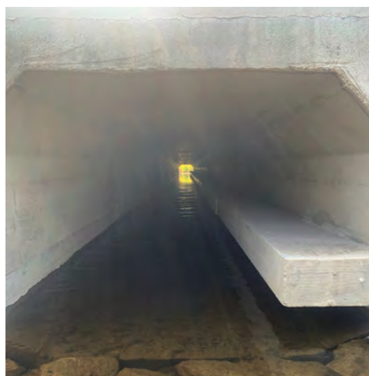
Completed culvert with integrated amphibian shelf
