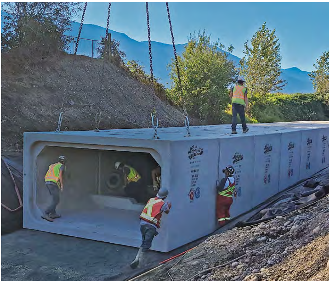
Installation of box culvert pieces
