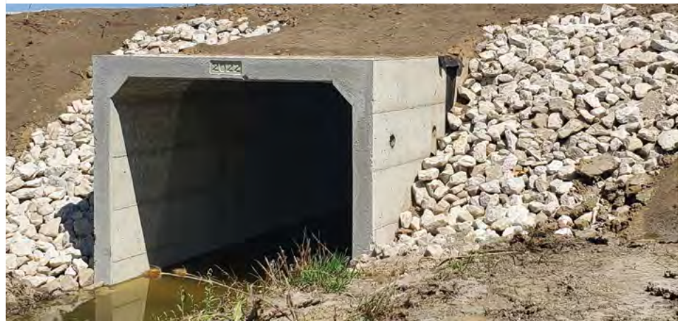
Installed precast concrete box structure
