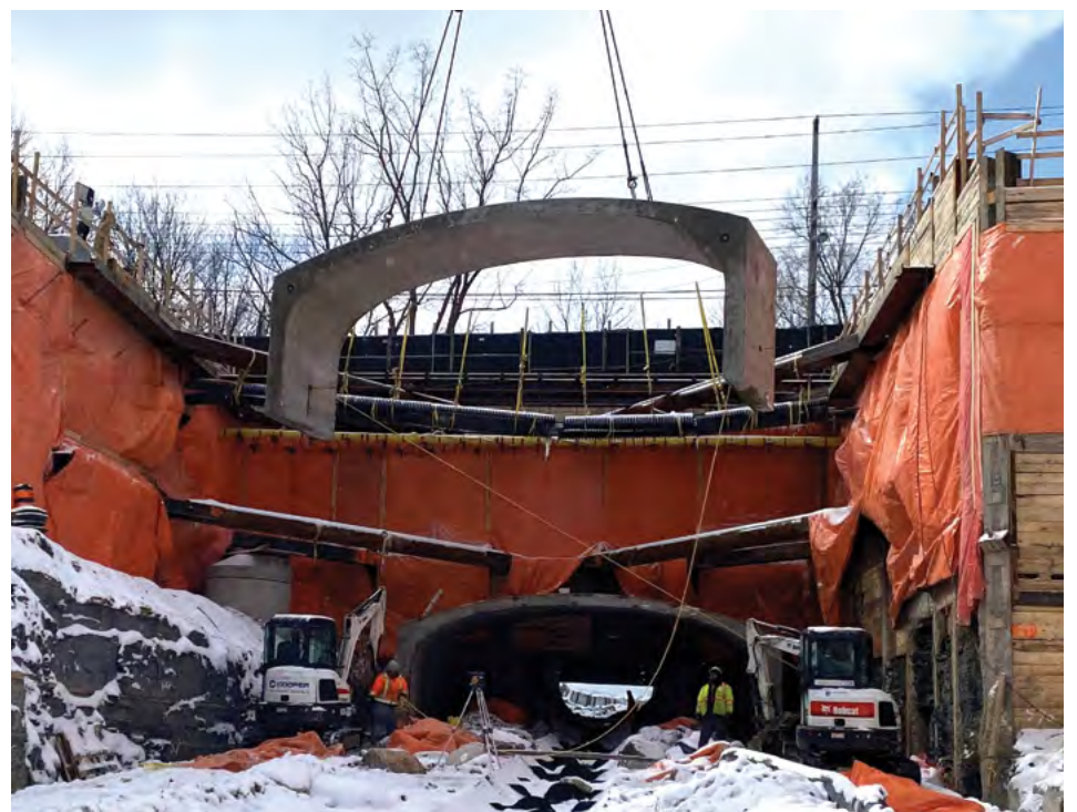
Lifting precast unit into place
