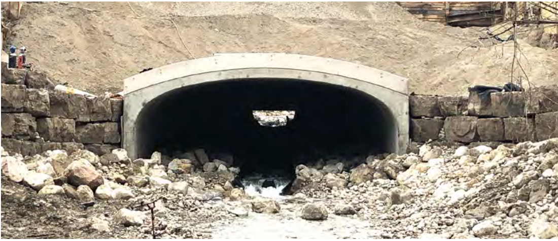
Placing backfill over completed structure
