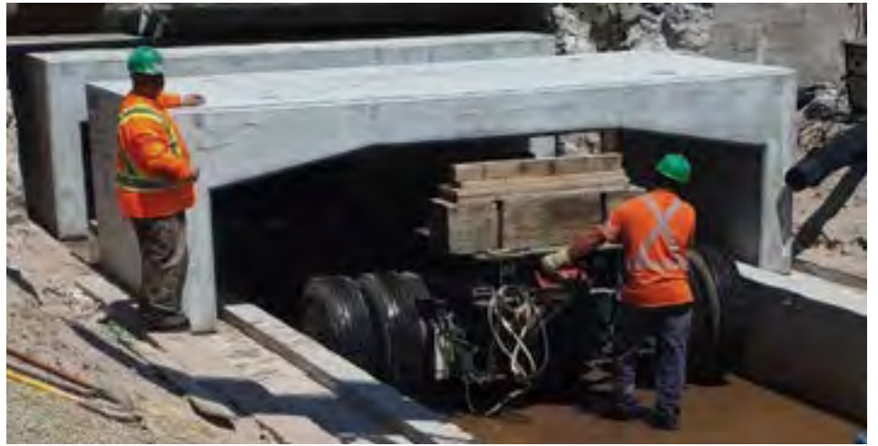
Hydraulic lift for open bottom culvert installation
