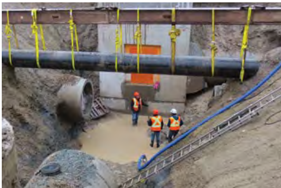
First half of lined chamber installed
