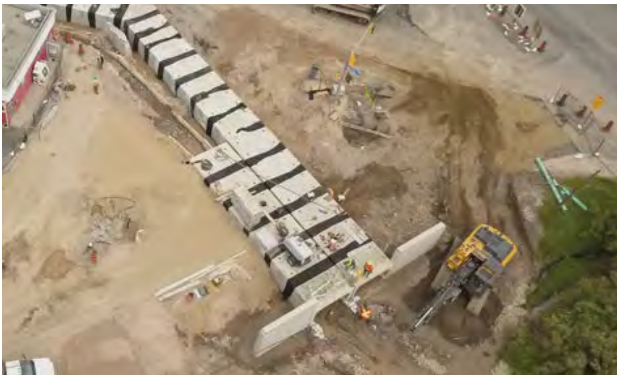
Fort Creek Aqueduct project aerial view
