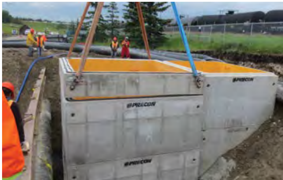
Last riser installed on lined chambers
