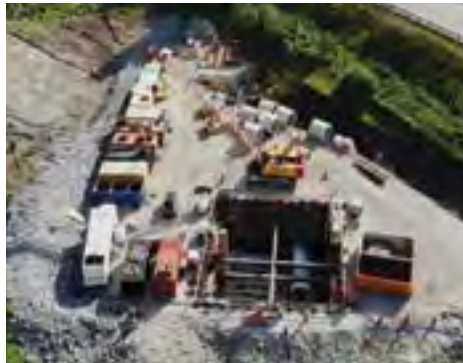
Aerial view of Highway 11 project
