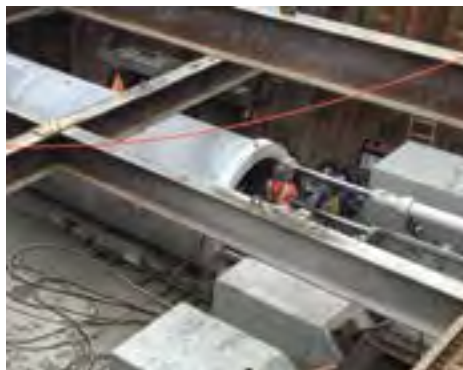
Launch shaft for microtunneling pipe
