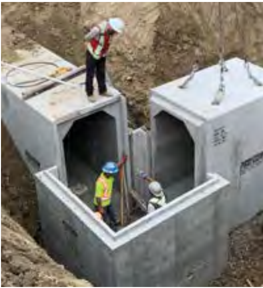
Maintenance hole and culvert connection
