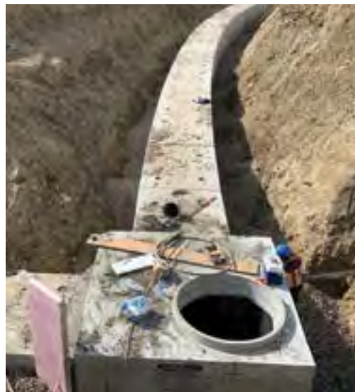
Box culvert designed and manufactured with a required radius
