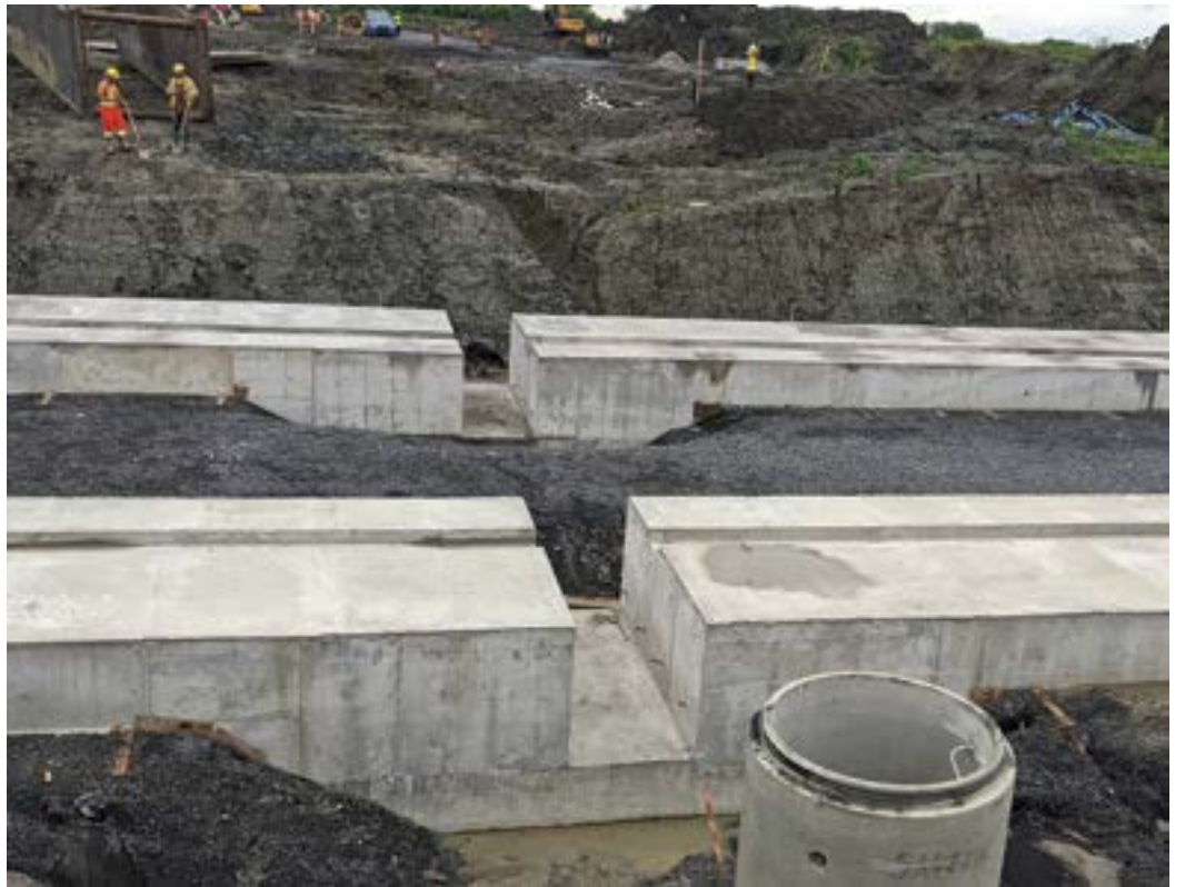
Gap in footing to allow for sanitary sewer installation
