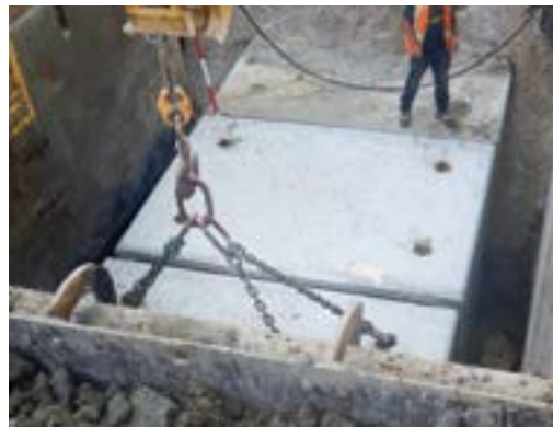
Box culvert installation
