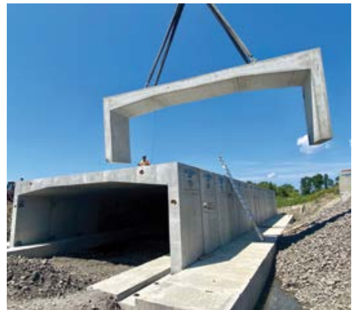
Open bottom culvert installation
