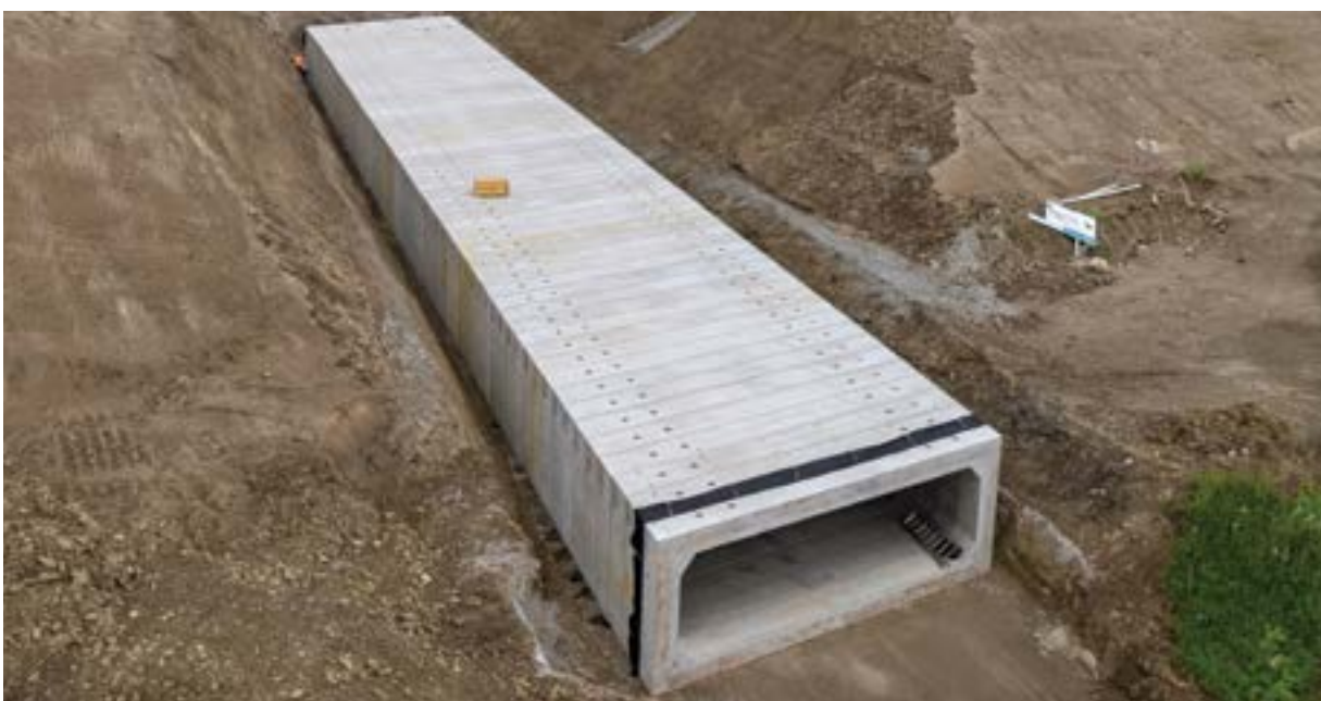
Completed installation of skewed box culvert
