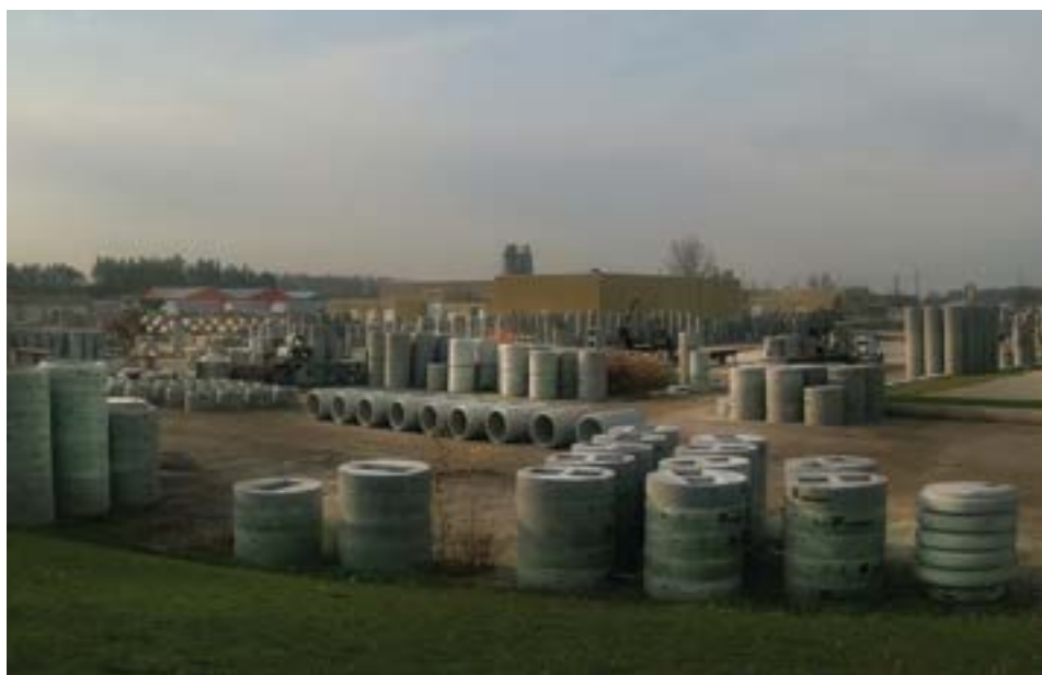
Forterra Pipe and Precast Manufacturing Plant – Cambridge, Ontario
