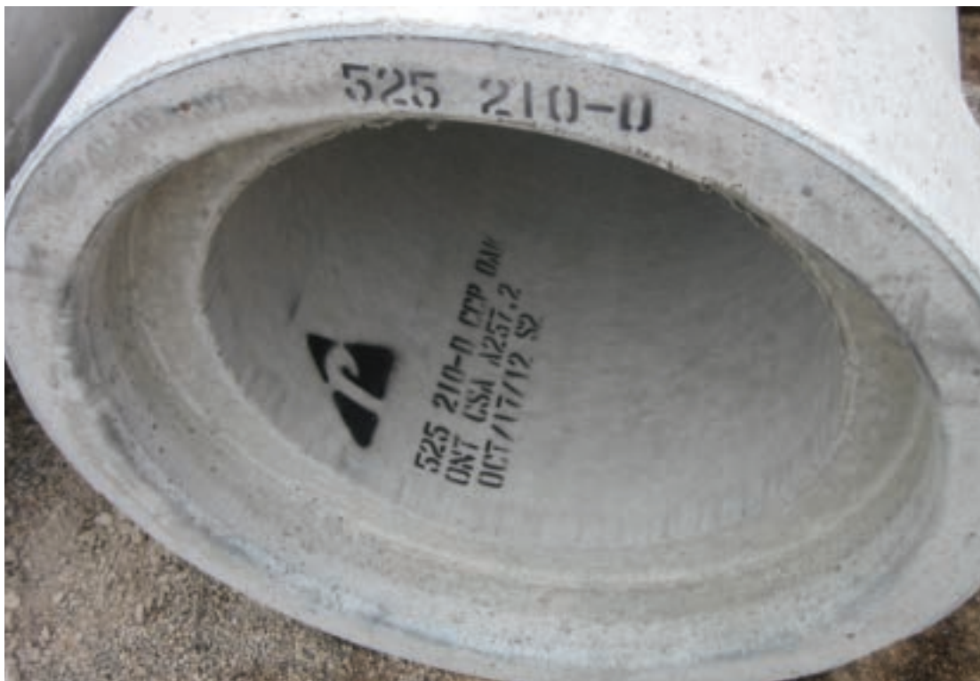
210-D class concrete pipe
