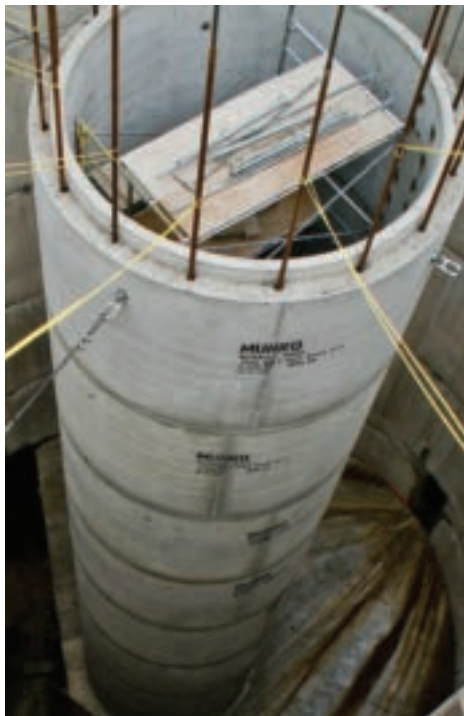
Pipe Tower Precast by Munro Ltd.
