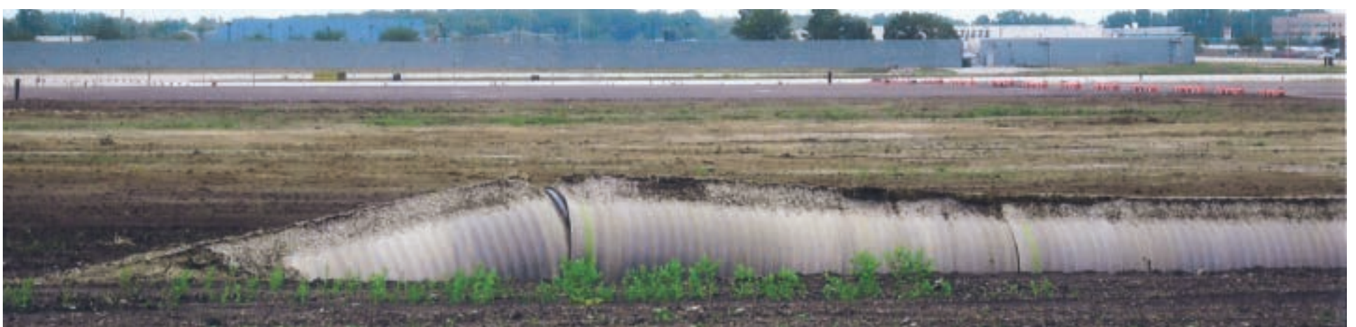
Floatation of 1,500mm diameter Polypropylene Pipe at Port Columbus International Airport
