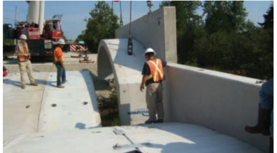
10.973m x 2.440m x 1.829m CON/SPAN unit being lowered into position
