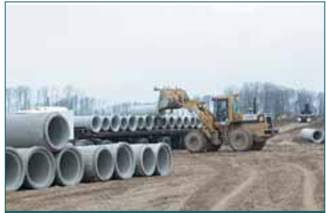
Handling Concrete Pipe
