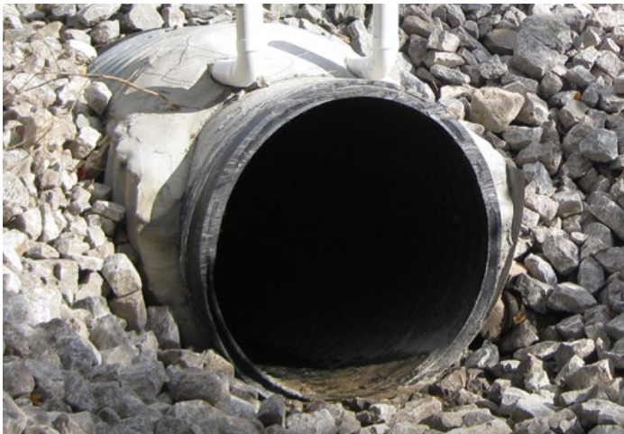
Relined culvert - reduced cross sectional area. This CSP culvert under Highway 407 in Ontario was relined after less than 20 years in service. The designer specified the appropriate rip rap protection to prevent erosion.
