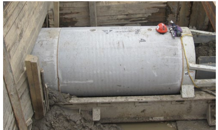
Jacking concrete pipe under Manitoba Highway
