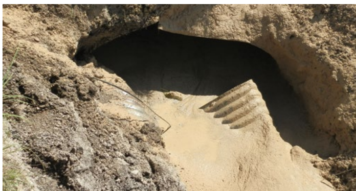
Decommissioned CSP culvert being filled with concrete
