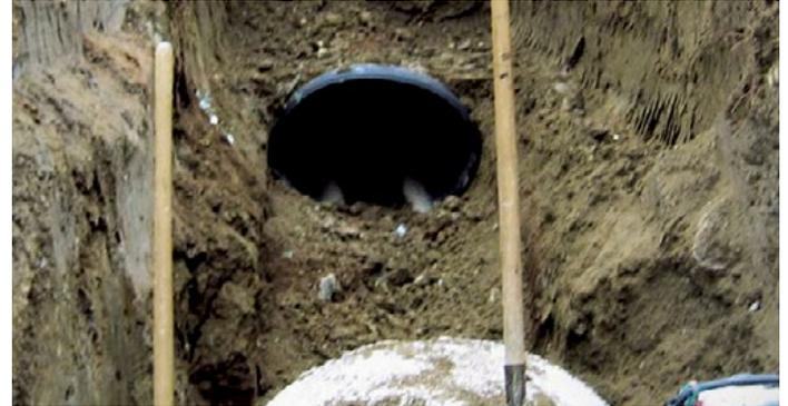
RCP being installed as HDPE is removed
